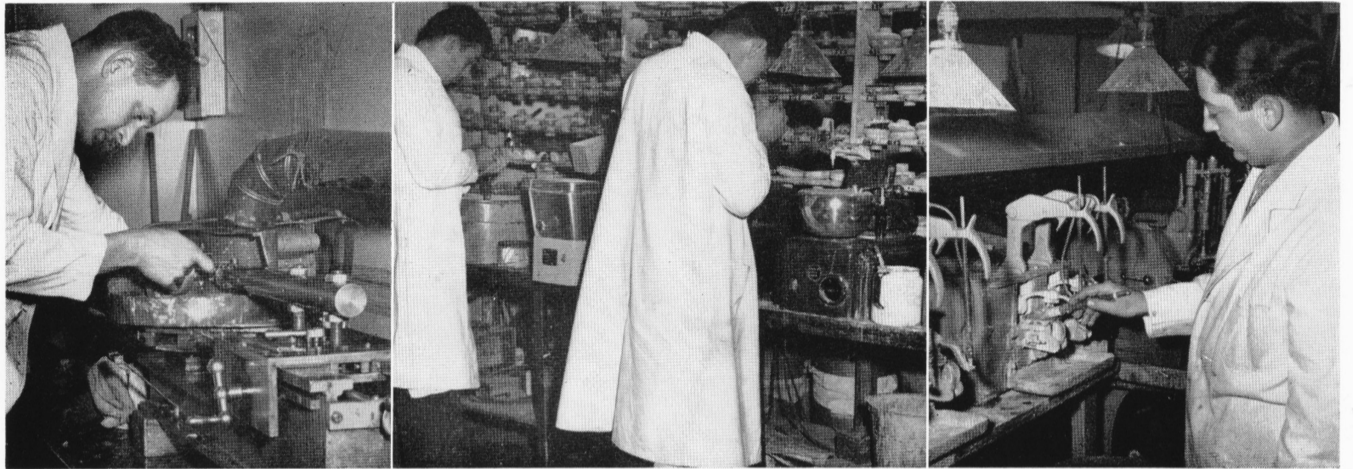
1) The diamond lap-operation: Bob Allen grinds the exact curve on the lens as required by the prescription. 2) The spherical finish and polishing, as applied by
